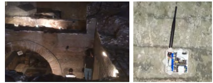
(b) Paper authors installing I/A devices.
